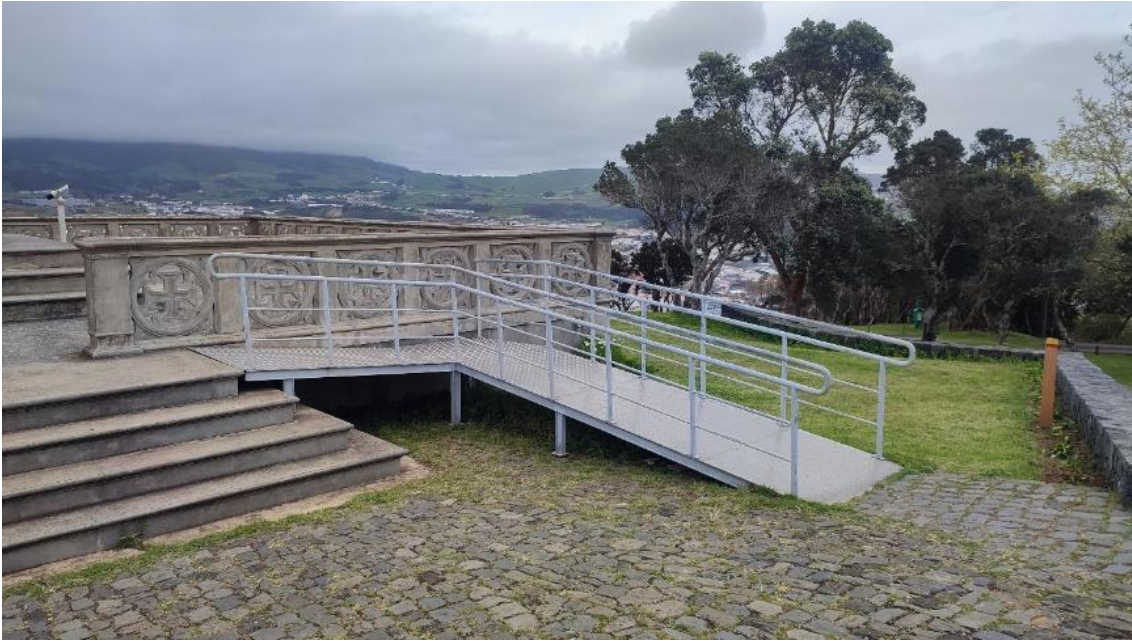
Figure 27. Ramp for users with reduced mobility at Pico das Cruzinhas viewpoint in Monte Brasil.
