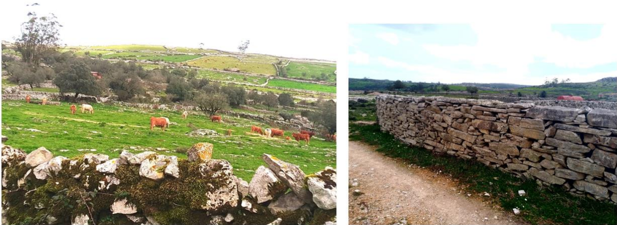
Figure 11. Dry stack stone walls in Sao Mamede. They serve various purposes such as fences, land demarcation, shelter or cows and for erosion control along the slope.
