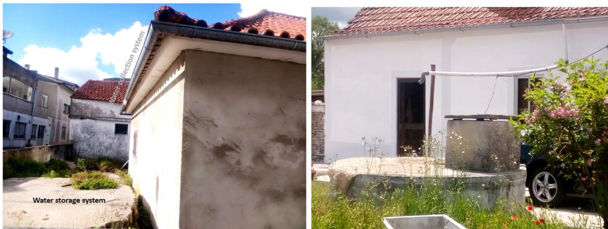
Figure 12. Rainwater harvesting system from different houses in Sao Mamede. The rainwater is collected from the roof and channeled to the storage system where the water is collected manually with rope and bucket.
