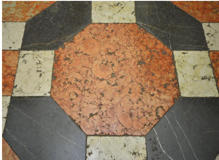
Figure 9. Tiles of red limestones with ammonites in the Camarín de la Virgen (Royal Monastery of Santa María de Guadalupe). These rocks come from Subbética (Córdoba Province) and are connection with the Sierras Subbéticas UNESCO Global Geopark.
